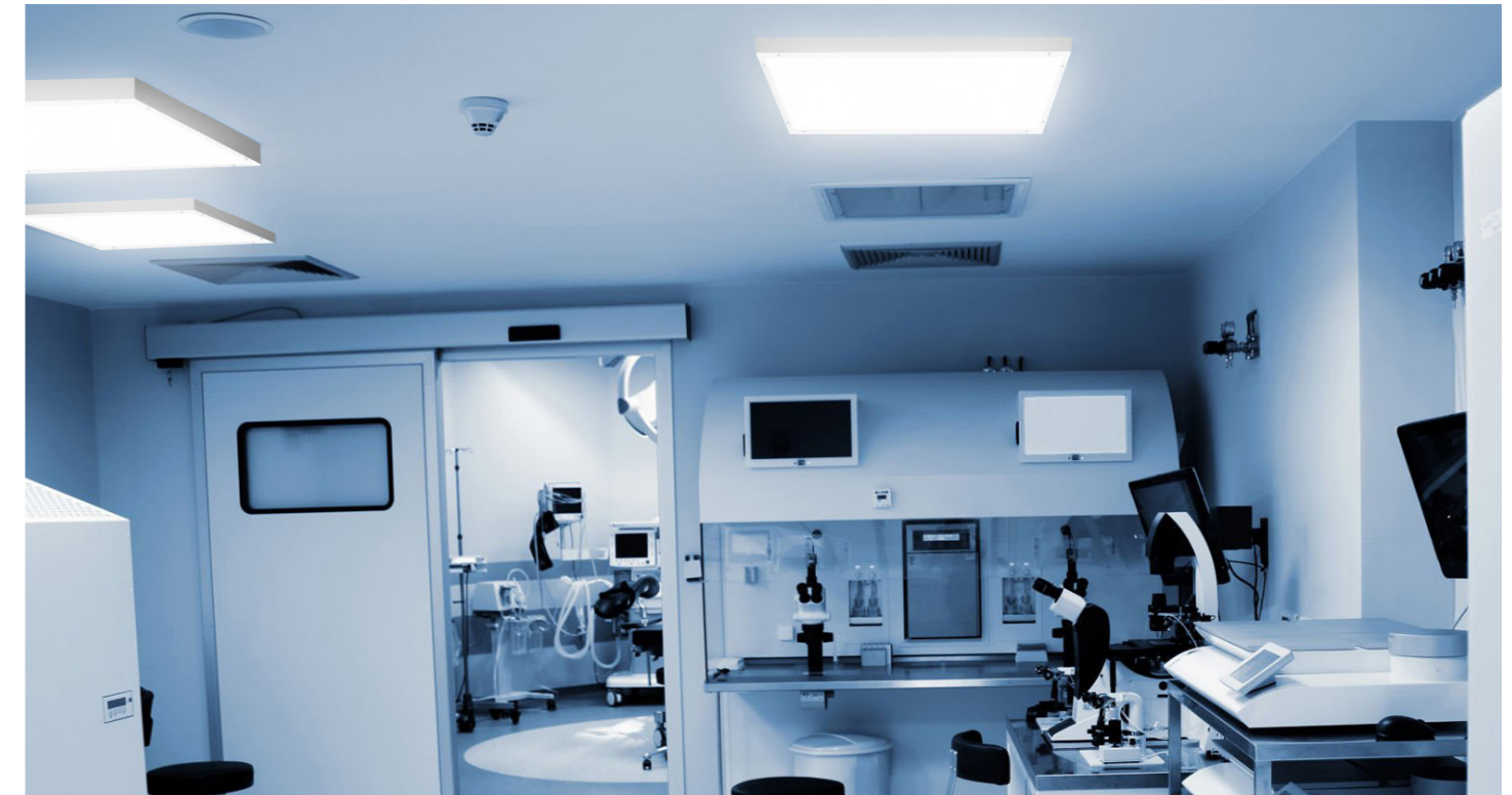
SALAS BLANCAS CLEAN ROOMS
